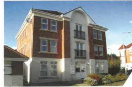
Deepcut £199,950 • Ground Floor Apartment • Two Bedrooms • Two Bathrooms • Kitchen • Lounge • Car Port Office tel: 01276 681682
