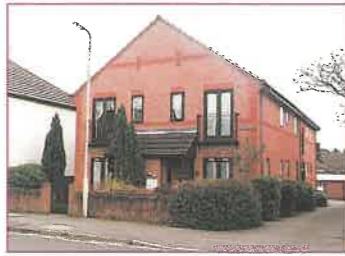
Fleet £89,950 CLARE/13289 A purpose-built apartment situated within close proximity of the town centre and mainline railway station. Entrance, bedroom 9'6" x 9'1", bathroom, lounge 13'9" x 12'6", kitchen 9'3" x 5'. Garage & parking. Apply: Fleet Office (01252) 620255
