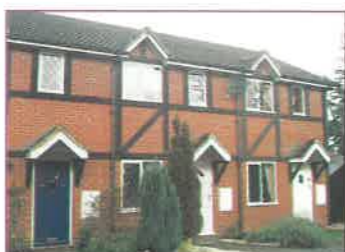
Lightwater £139,950 THEOR/13108 A mid-terrace property situated on the Lightwater Grange development. Entrance, lounge 12'3" x 13'5" max., kitchen 12'3" x 10'6". Landing, bed 1 12'3" x 10'5", bed 2 10'2" x 6'8", bathroom. Rear garden approx. 44' deep. Apply: Lightwater Office (01276) 452000
