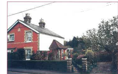
West End, Woking £219,950 GLADS/13422 A semi-detached cottage in need of modernisation, situated in a non-estate location. Entrance, lounge 13'7" max x 12'3" max, dining room 12'2" max x 11'7" max, kitchen 11'5" x 8'6", bathroom, separate w.c. Landing, bedroom 1 11'7" x 11'3", bedroom 2 12'2" x 11'7" max. Rear garden approx. 60' x 42', off-street parking. Apply: West End Office (01483) 797974
