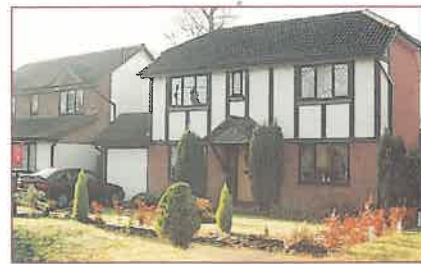
Farnborough £179,950 WOODL/12706 A detached property situated in a cul-de-sac location. Entrance hall • cloakroom • kitchen/breakfast room 16' x 9'11" • living room 16' x 11'2" • conservatory 12'11" x 10'11". Landing • bed 1 12'6" max. into recess x 10' • en-suite • bed 2 11'3" x 9' • bed 3 8'2" x 6'7" • bathroom. Rear garden • garage. Apply: Farnborough Office (01252) 370008
