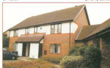
FLEET A ground floor apartment in a cul-de-sac position with double glazed windows. Entrance porch, lounge 18' x 10', kitchen 8'6 x 6'7, inner hallway, bedroom 1 11'5 x 9'8, bedroom 2 9'6 x 8'2, bathroom. Parking, carport and communal grounds. Available with no onward chain. Price: £115,000 Apply: Fleet Office (01252) 620255
