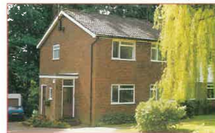
CAMBERLEY A ground floor maisonette situated approximately two miles from Camberley town centre and railway station. Entrance hall, sitting room 14' x 10', re-fitted kitchen 11'3 x 6'7, bedroom 1 10'6 x 10', bedroom 2 11'4 x 7'1, re-fitted bathroom. Garage, established communal grounds. Price: £129,950 Apply: Camberley Office (01276) 22088
