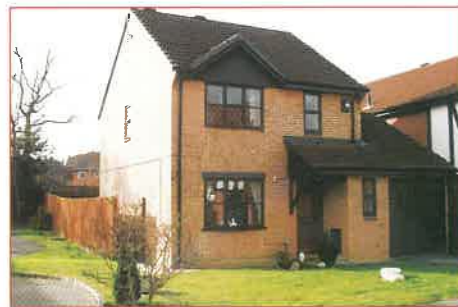
BAGSHOT A detached Heron built 'Viscount' style property with re-fitted en-suite shower room and re-fitted bathroom. Entrance hall, cloakroom, living room 14'1 x 11', dining room 10'2 x 8'10, kitchen 11'4 x 9'1, utility room 7'2 x 6'1. Landing, bedroom 1 14'7 x 8'5, en-suite shower, bedroom 2 11'6 x 9'3, bedroom 3 7'9 x 6'6, re-fitted bathroom. Rear garden approx. 36' in depth x 30', garage.
