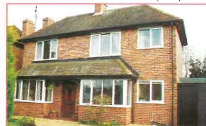
CAMBERLEY Double glazed windows, re-fitted kitchen and re-fitted bathroom. Entrance hall, sitting room 13'6" x 10'6", dining room 14'6" max. x 10'6" max., fitted kitchen 12' x 6'. Landing, bedroom 1 14'10" max. x 9'5" max., bedroom 2 11' max. x 10' max., bathroom. Rear garden approx. 42' x 15'.
