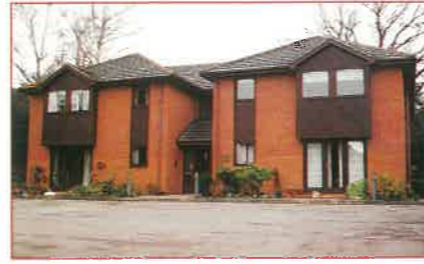
LIGHTWATER A one bedroom first floor retirement apartment set in communal grounds with communal parking. Entrance hall, living room 15'10" x 14'8" max., kitchen 12'10" max. x 6'6", bedroom 15' x 9'2", bathroom.
