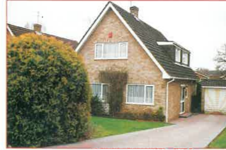
LIGHTWATER A three bedroom detached house. Entrance hall, cloakroom, living room 22'1 x 11'8, dining room 11' x 11'6, conservatory 8'6 x 11'6, kitchen/breakfast room 21' x 10', bedroom 1 14'2 x 11'8 max., bedroom 2 12'2 x 10'10, bedroom 3 12'2 max. x 7' max., bathroom, garage, garden approx. 42' in length.
