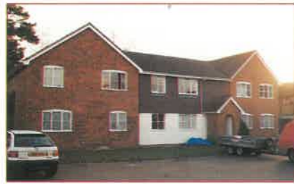
BAGSHOT A first floor Charles Church 'Richmond' style flat situated on Connaught Park. Entrance door leading to: lounge/kitchenette 18' max. x 11'9", bedroom 11' x 10', bathroom. Outside: communal grounds and communal parking.
