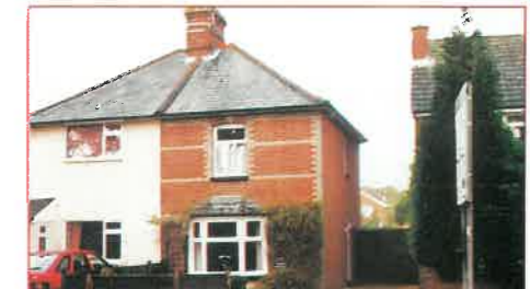
CHURCH CROOKHAM A turn of the century semi-detached cottage with a 55' approx. rear garden. Front door to: dining room 14' x 11'9", living room 13'4" x 13'2", kitchen 11'2" x 6', bathroom, separate w.c. First floor, landing, bedroom 1 12'2" x 11', bedroom 2 12' x 9'2". Garden approx. 55' in length, gravel driveway.
