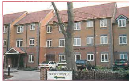
CAMBERLEY A first floor self-contained flat available to purchasers of 60 and over. Lift, residents living room, laundry room and guest suite. Entrance hall, sitting/dining room 23'6 (max.) x 10'8 (max.), kitchen 7'7 x 7', bedroom 17'4 (max.) x 9'4 (max.), bathroom. Price: £74,000 Apply: Camberley Office (01276) 22088
