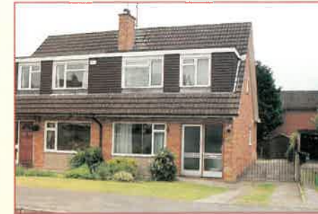
GLOUCESTER ROAD, BAGSHOT
