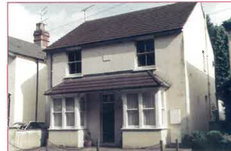
CAMBERLEY A ground floor maisonette with two double bedrooms situated within half a mile of Camberley town centre and railway station. Covered entrance porch, entrance hall, sitting room 13' (max.) x 10'5, conservatory 9'1 x 7', kitchen/breakfast room 11' x 10'4, bathroom, bedroom 1 14'8 into bay x 10'6 (max), bedroom 2 14'8 (max) x 10'6 (max). Outside: front garden, rear garden 57' long (min) x 25' wide (min)
