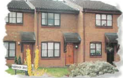
CAMBERLEY £84,950 Situated in Cheylesmore Park. Living room 16'2" x 11'8", kitchen, 2 beds., bathroom. 35' rear garden. Apply: Camberley Office (01276) 22088
