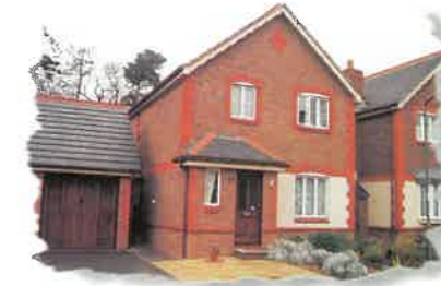
CAMBERLEY £159,950 Detached 'Cala' home. Cloakroom, lounge, dining room, kitchen, utility area, 3 beds., en-suite shower, bathroom. Garage, garden. Apply: Camberley Office (01276) 22088
