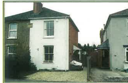
LIGHTWATER £99,950 A turn of the century semi detached cottage. Entrance hall, lounge 12' (max) x 11'4", dining room 12' x 12' (max), kitchen 14' x 6'9", bathroom, landing. Bedroom (1) 12' (max) x 11'3", (2) 12' (max) x 11'3", garden. (Apply Lightwater Office)
