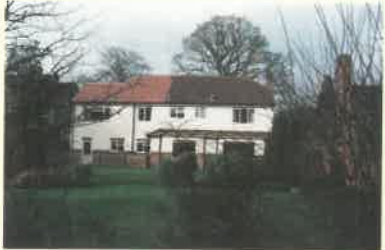
View from the rear boundary
