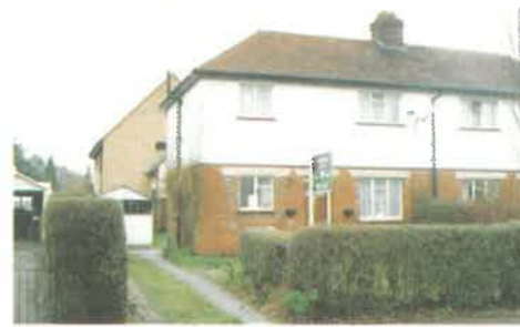
THE AVENUE A semi-detached house with a re-fitted bathroom. Living room 15'10 x 11'6, kitchen 10'10 x 8'8. Two bedrooms. Garage. £64,950
