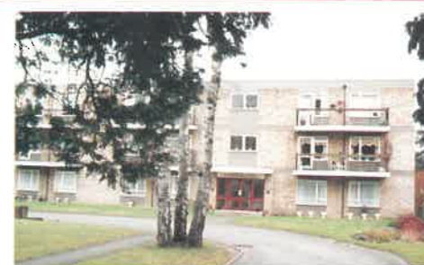
UPPER PARK ROAD A first floor flat. Lounge/dining room 25' x 13', kitchen 11'1 x 8'. Two bedrooms, bathroom. Communal grounds, garage. £75,000
