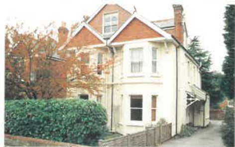
UPPER GORDON ROAD A ground floor flat. Lounge 16'9 x 11'10 (max), kitchen 10'8 x 7'10, bedroom, bathroom, separate w.c. Garden, parking. £54,950
