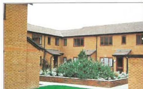
KIRKBY COURT From £53,950 A brand new development of one bedroom flats, situated close to Frimley town centre. Features include NHBC warranty, double glazing, gas radiator central heating, fitted kitchen with gas hob, electric oven and cooker hood.
