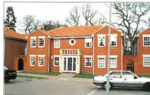
LE MARCHANT ROAD £81,950 A ground floor apartment with en suite bathroom, garage and garden. Lounge/dining room 20'10 x 20'5 (max), kitchen 8'6 x 6'11, bedroom (1) 14'1 x 9'8, en suite bathroom, bedroom (2) 14'1 x 6'7, shower room. Garage, garden.
