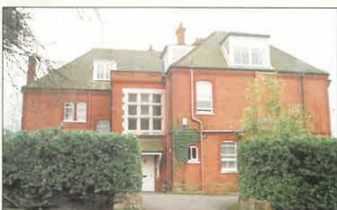
HEATHERDALE ROAD £59,950 A Victorian ground floor maisonette which requires some updating, in attractive communal grounds. Cloakroom, sitting room 15'3" x 13'10" (max), kitchen 10' x 5'11", bedroom (1) 15' (max) x 8'4", bedroom (2) 11'3" x 9'4", bathroom. Communal gardens, garage.
