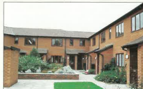
PARSONAGE WAY From £53,950 A brand new development of one bedroom flats, situated within walking distance of Frimley town centre. The specification includes NHBC guarantee, double glazing, gas radiator central heating, kitchen with appliances and allocated parking.
