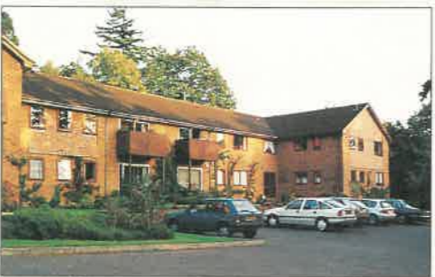
COLLINGWOODRISE £89,950 & £95,000 A choice of first floor or ground floor apartments with two bedrooms, in an exclusive development. Features include light oak fitted kitchens, en suite shower room and additional bathroom, garage and well tended communal grounds. Offered for sale with no chain involved.
