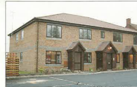
YORK ROAD £49,750 A brand new development of one bedroom flats with luxury kitchens and bathrooms, double glazing, NHBC guarantees and many other features, situated within walking distance of Camberley town centre.
