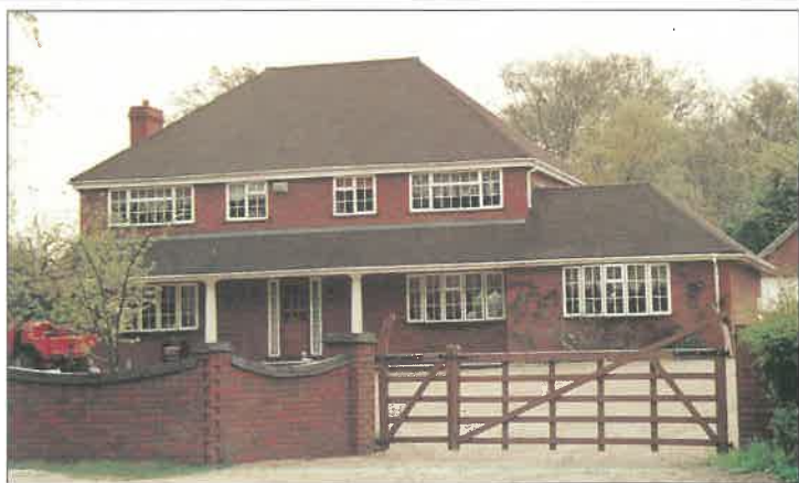
BAGSHOT London Road A Georgian style property on the outskirts of Bagshot. Living room 24'9 x 15'6, study 11'4 x 11', family room 17'2 x 16'2, kitchen/breakfast room 13'5 x 11'9, utility, dining room 12'9 x 10'5, shower room Bedroom (1) 17'4 x 10'4, en-suite bathroom, (2) 12'3 x 12', (3) 12'10 x 10'10, (4) 11'6 x 11'2, bathroom. Gardens, double garage. £250,000 Sole agents
